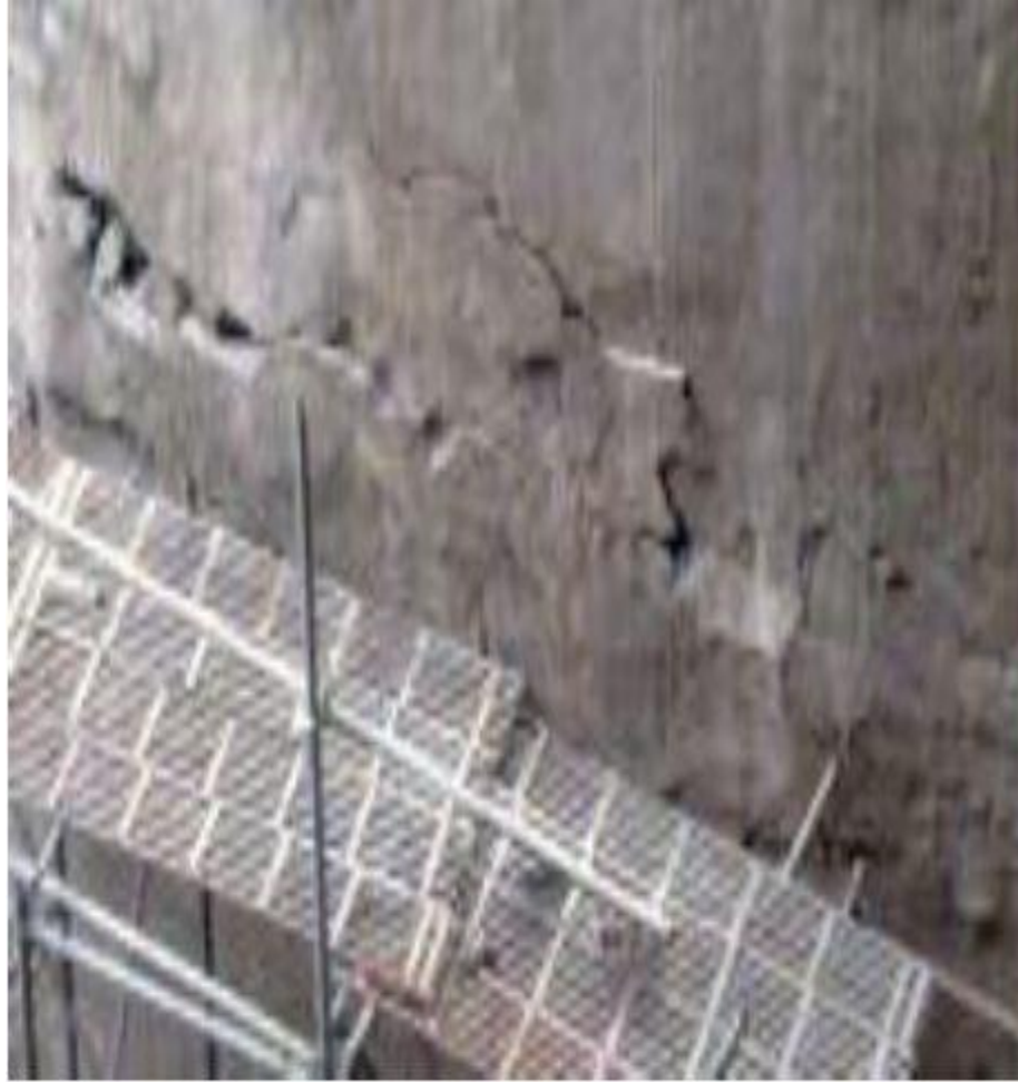
Silo wall crack before and after chipping the concrete. Comment on the nature of the cracks.
