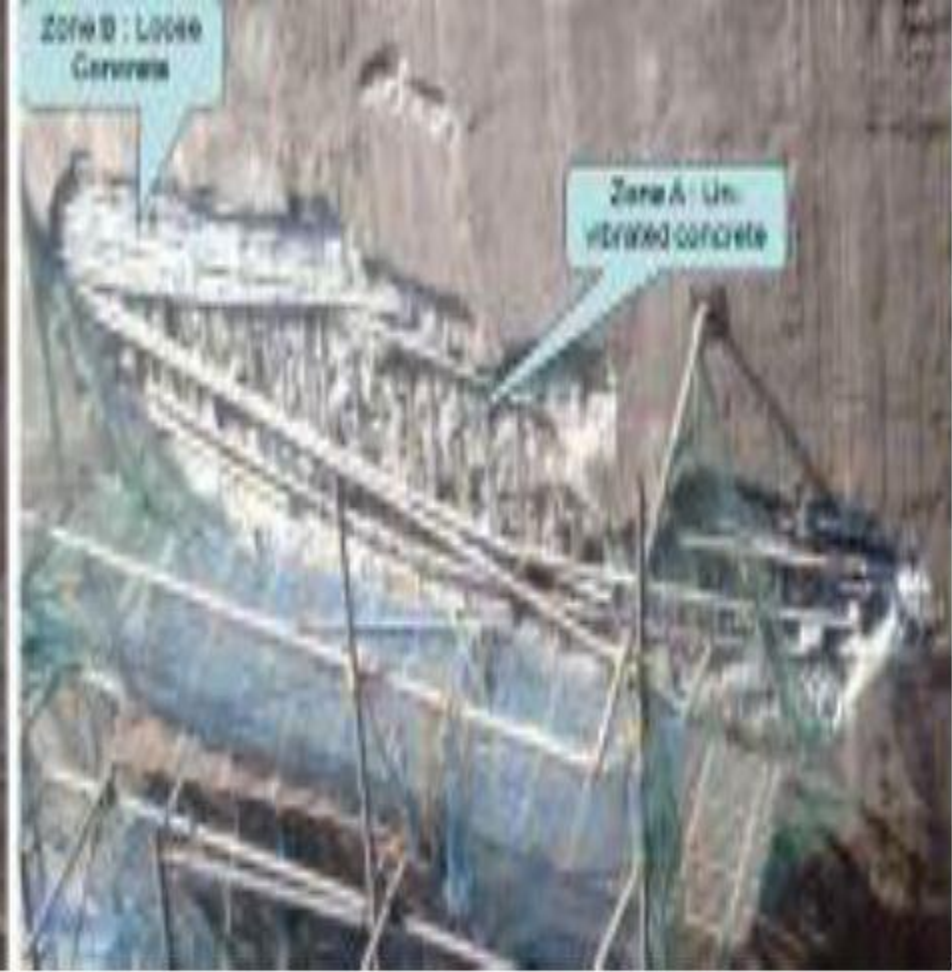
Silo wall crack before and after chipping the concrete. Comment on the nature of the cracks.
